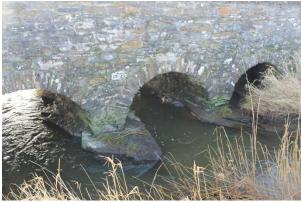
Figure 6 a) bridge along Dounby transect showing piers founded on bedrock, b) stream channel cut into bedrock.
